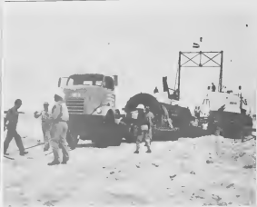
THIS OPERATION takes on all the aspects of a World War II invasion as heavy equipment rolls off the ramp of a landing craft. In actuality, it's the delivery of a 120-ton ammonia converter on the beach at Barracuda for the Antilles Chemical Company's plant.
